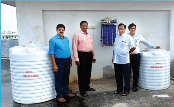
Providing R.O. Water Purifier system to Oxford Public School, Guntur
