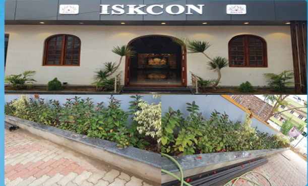
Setting up Public Park at ISKCON Temple Campus at Vijayawada.
